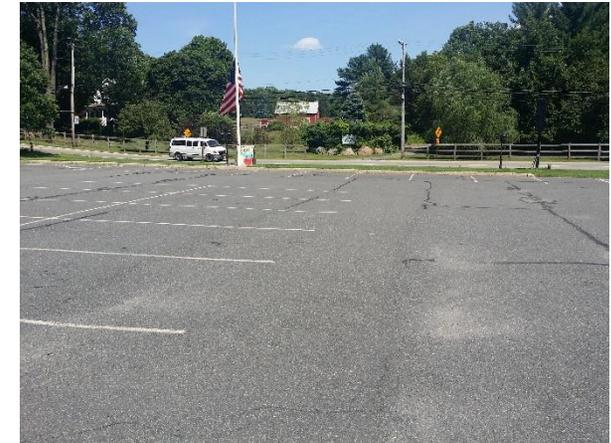
A large amount of runoff is generated from Howard Boulevard during storm events. A bioretention system can be implemented in the grass area along the road, and a curb cut will allow this system to capture, treat, and infiltrate stormwater runoff before it reaches the catch basin. A preliminary soil assessment suggests that the soils have suitable drainage characteristics for green infrastructure.
