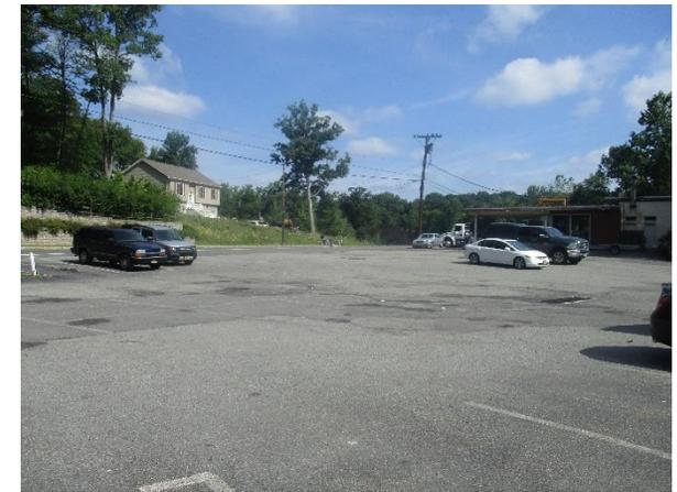
Stormwater from the rooftops of Vinny & Sons Pizza and Bagel Mike's building runs directly onto the parking lot. The parking spaces along the building can be replaced with pervious pavement to allow water to infiltrate through the surface. A preliminary soil assessment suggests that the soils have suitable drainage characteristics for green infrastructure.
