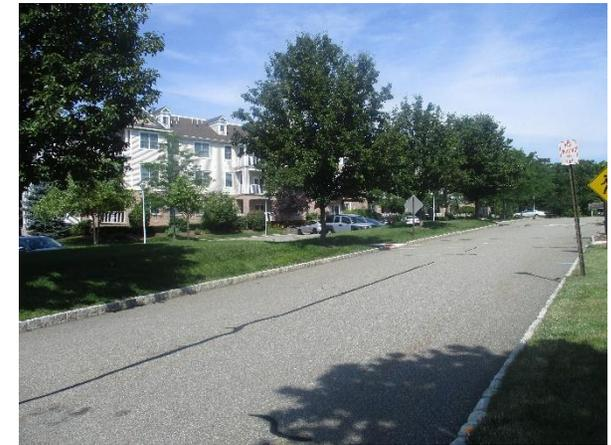
A large amount of runoff is generated by the parking lot and the buildings during storm events. Sections of parking spaces can be replaced with pervious pavement to capture, treat, and infiltrate runoff from roofs and the parking lot. Rain gardens can be implemented in the grass islands and alongside buildings. A preliminary soil assessment suggests that the soils have suitable drainage characteristics for green infrastructure.
