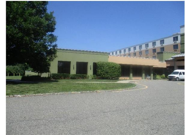
A large amount of runoff is generated by the parking lot during storm events. Most of the parking spaces can be replaced with pervious pavement to efficiently manage this stormwater runoff. Two rain gardens can be installed in the grass area along the west side of the building to capture, treat, and infiltrate stormwater runoff from the driveway. A preliminary soil assessment suggests that more soil testing would be required before determining the soil's suitability for green infrastructure.
