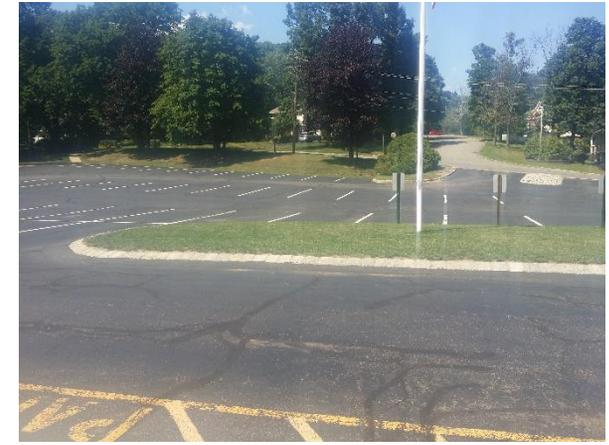
A large amount of runoff is generated by the parking lot during storm events. Multiple strips of parking spaces can be replaced with pervious pavement to capture and infiltrate stormwater. Additional runoff can be managed by implementing a rain garden in the island located in the front parking lot. A preliminary soil assessment suggests that the soils have suitable drainage characteristics for green infrastructure.
