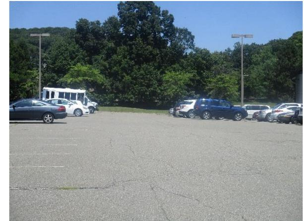
A large amount of runoff is generated by the parking lot during storm events. Most of the parking spaces can be replaced with pervious pavement to efficiently manage this stormwater runoff. A preliminary soil assessment suggests that more soil testing would be required before determining the soil's suitability for green infrastructure.
