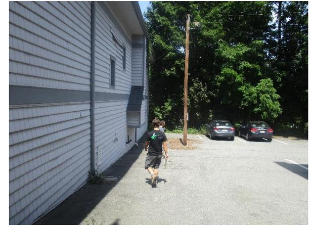
A large amount of runoff is generated by the parking lot during storm events. The parking spaces farthest from the building can be replaced with pervious pavement to allow water to infiltrate through the surface. A preliminary soil assessment suggests that the soils have suitable drainage characteristics for green infrastructure.
