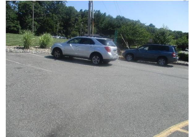
A large amount of runoff is generated by the parking lot during storm events. Parking spaces along the west and south sides of the building can be replaced with pervious pavement to manage this stormwater runoff. A preliminary soil assessment suggests that the soils have suitable drainage characteristics for green infrastructure.
